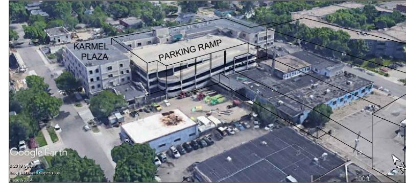
6 AERIAL VIEW - SOUTHWEST CORNER A1.2 NO SCALE
