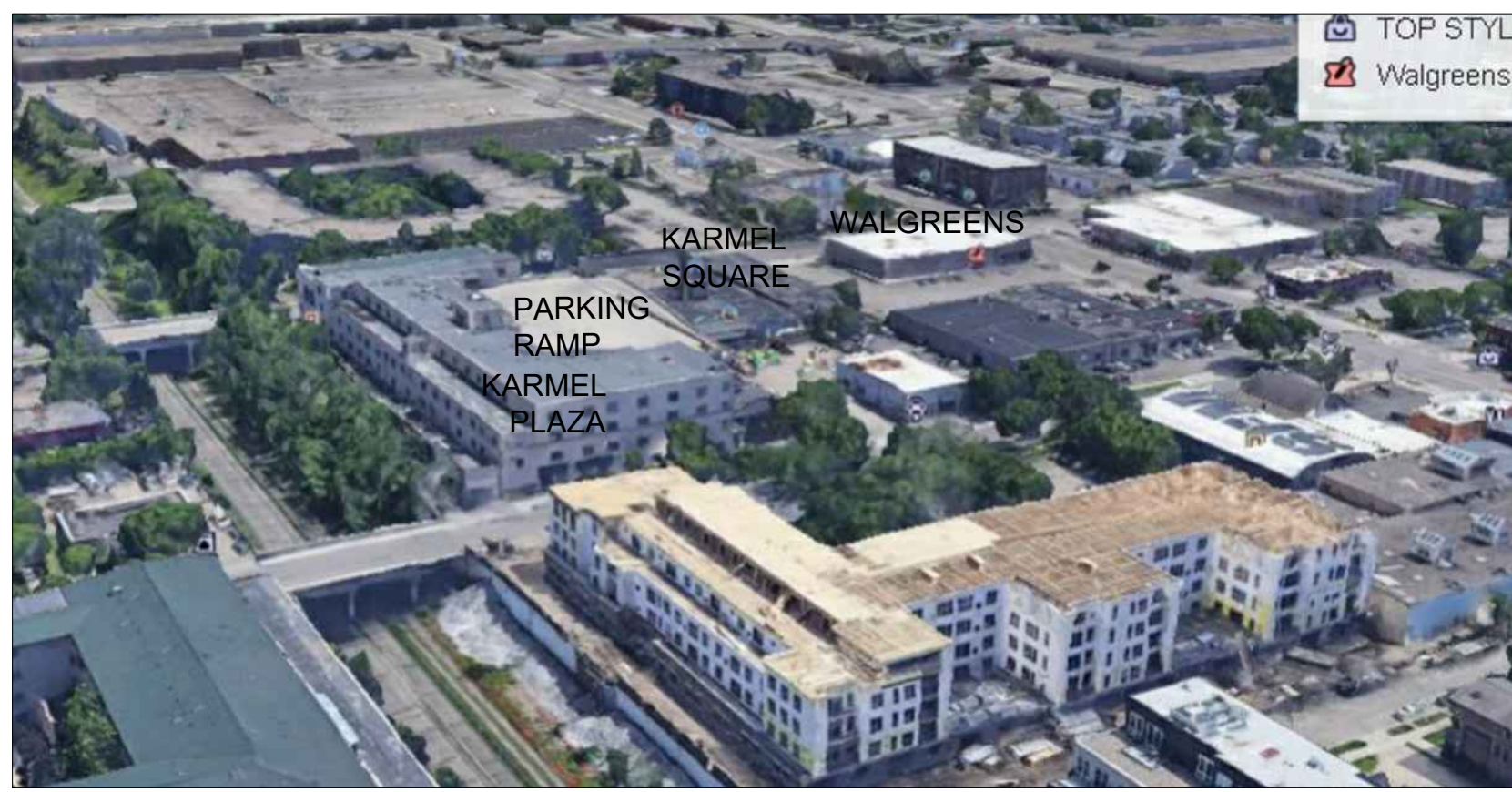
2 AERIAL VIEW - NORTHWEST CORNER NO SCALE
