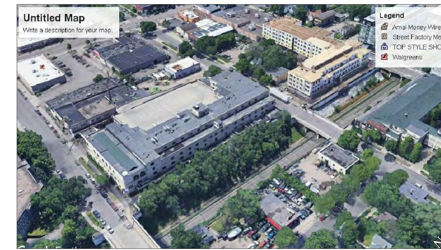
9 AERIAL VIEW - NORTHEAST CORNER NO SCALE
