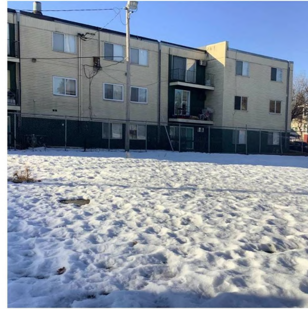
New Building Site Looking SW at Adjacent Building
