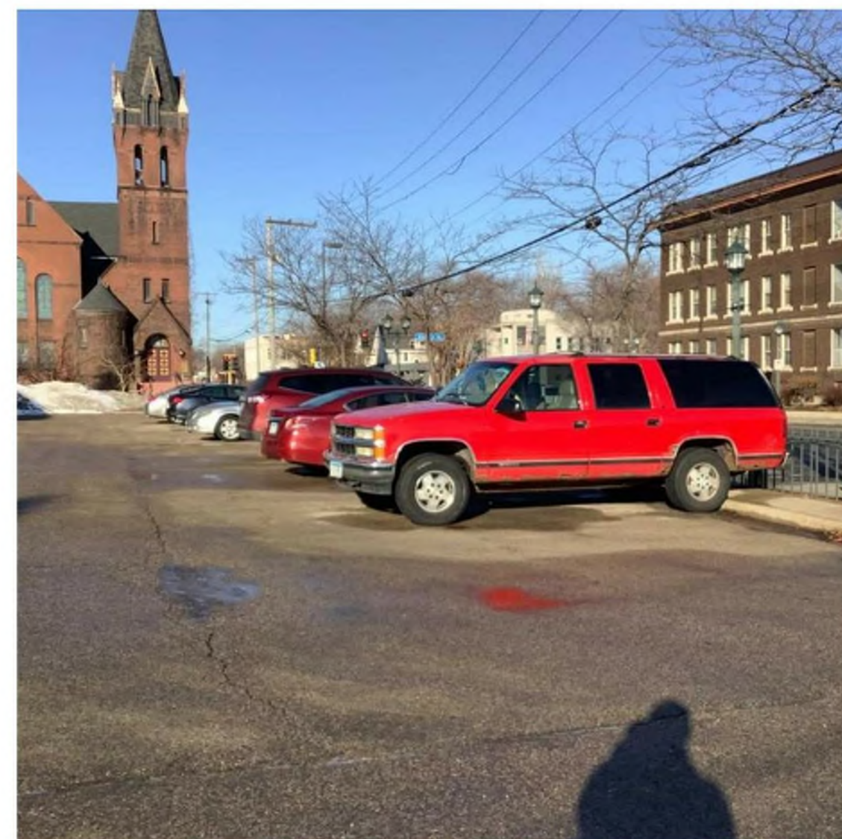
Existing Parking Lot Looking NW
