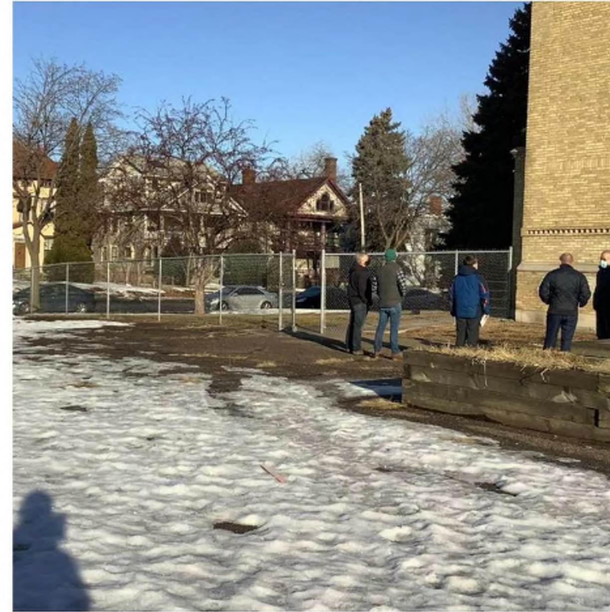
New Building Site Looking NW
