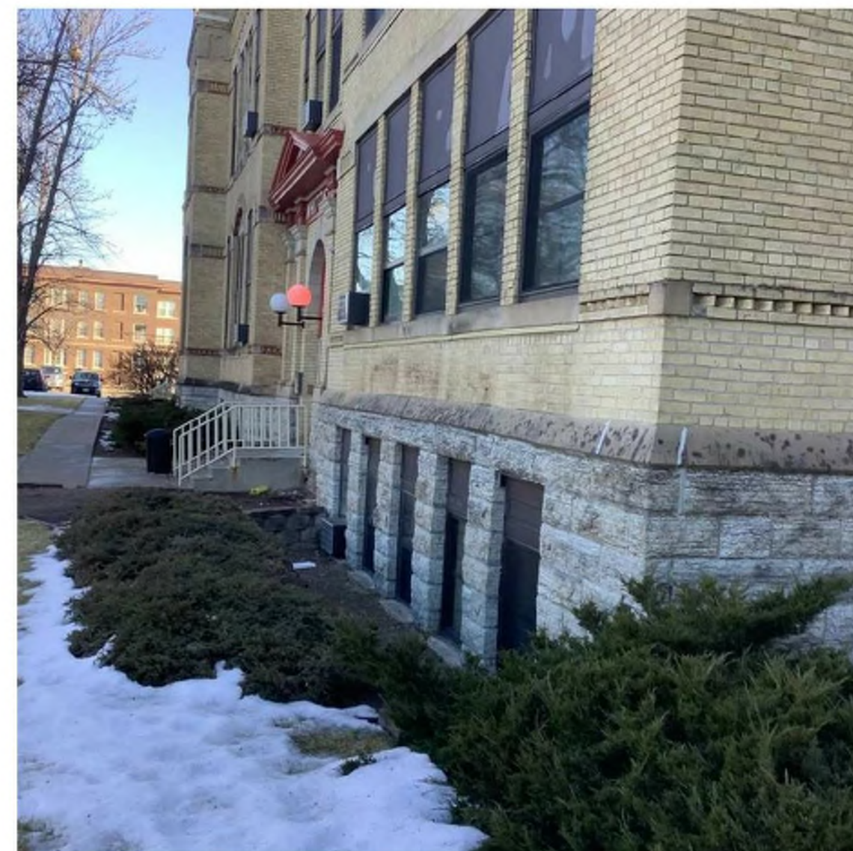
Front of Existing Building Looking North
