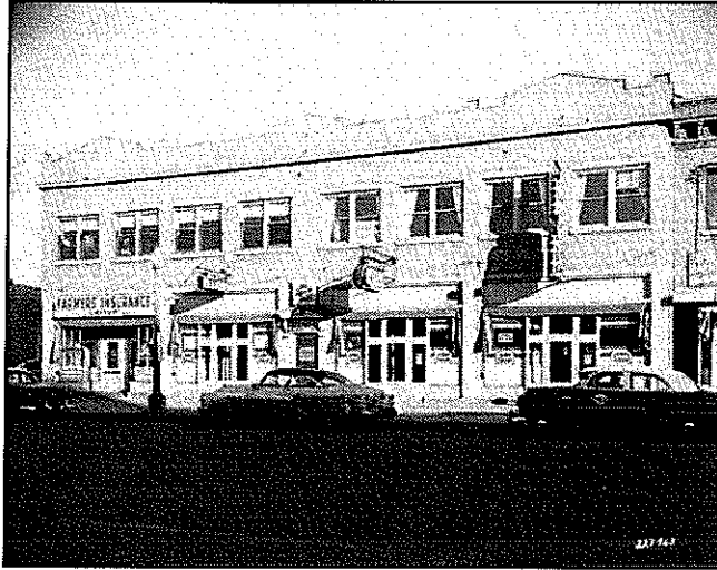
Business block with the USS Yorktown VFW Post, 2947-1/2 Lyndale, 1955, later renovated into the Jungle Theater (Norton and Peel, photographer; Minnesota Historical Society)
