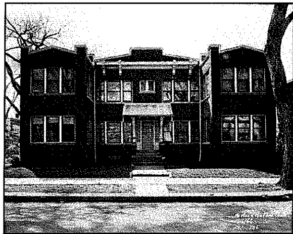
Apartment Building, 2322 Garfield, 1966 (Norton and Peel, photographer; Minnesota Historical Society)
